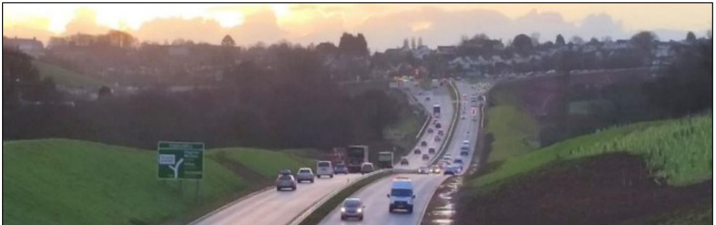
Figure 17: South Devon Link Road completed scheme
